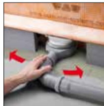
=> 5. Ajuster le tuyau d'évacuation
