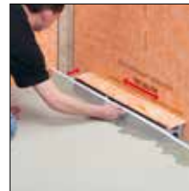
=> 4. Ajuster le support de caniveau
